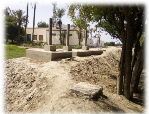
Sewerage Treatment Unit (STU)
