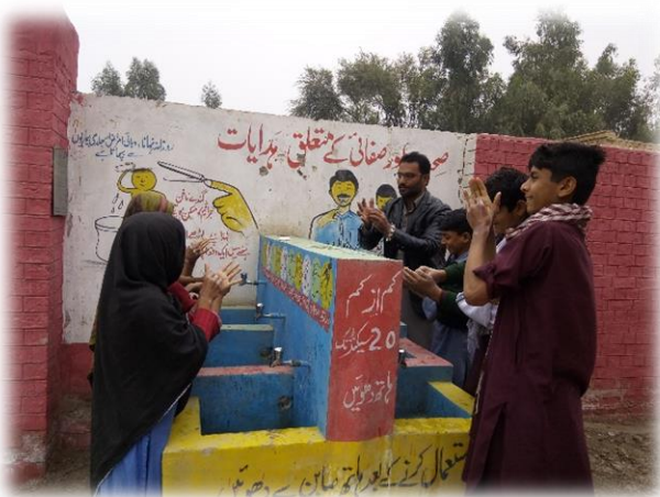
Group Handwashing Station
