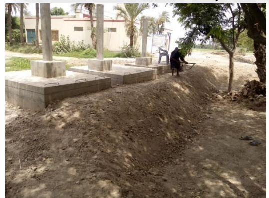
Sewerage Treatment Unit (STU)
