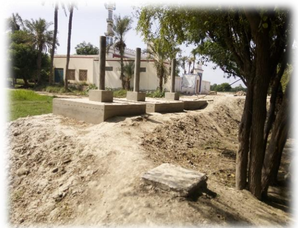
Sewerage Treatment Unit (STU)
